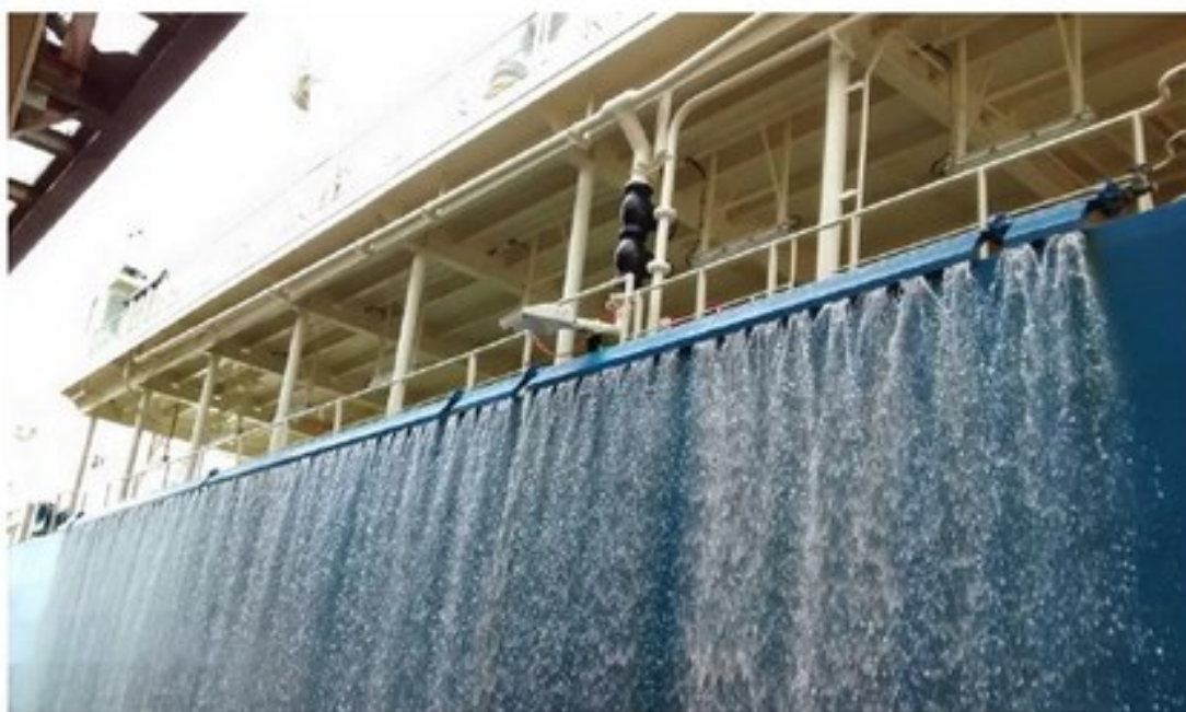
Plate 2-5: Water curtain use during LNG transfer (Source: Ian Lawson and Nicholas Ratinaud)
